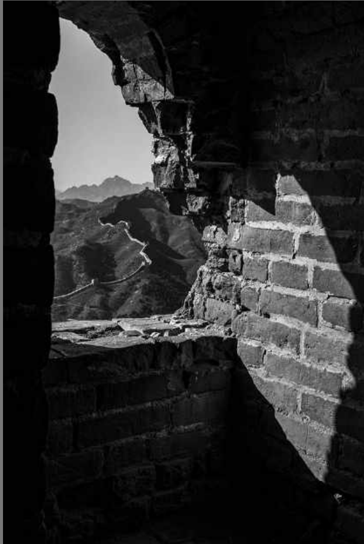
“CRACK AT THE GREAT WALL” by BOB CHIU
